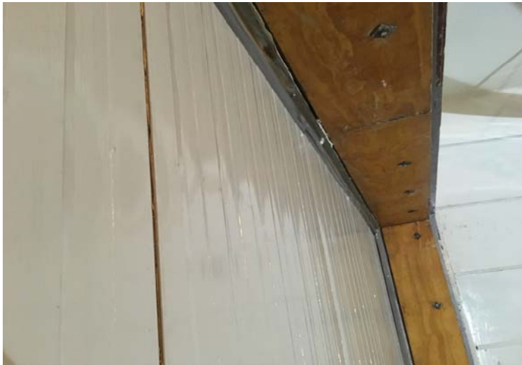
Figure 3: Interior side of roof panels in test rooms
