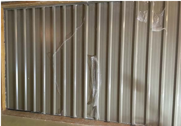
Figure 4: Exterior side of the roof panels showing corrugations
